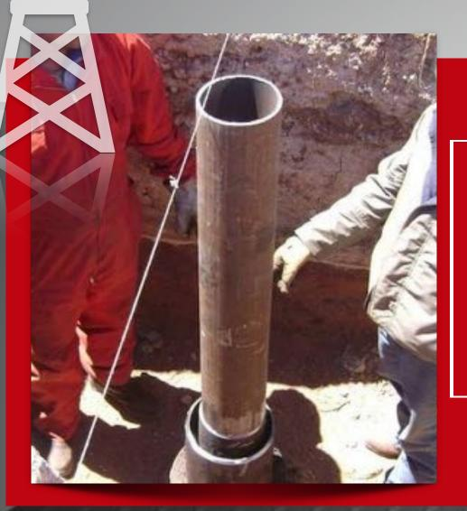
THE 7" CASING EXTENSION IS READY TO BE WELDED TOGETHER
