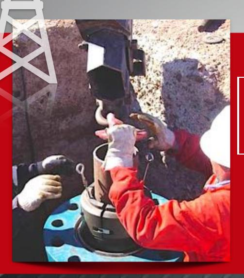
THE PACKER IS PLACED IN THE ANULUS OF THE 9 5/8" WELLHEAD
