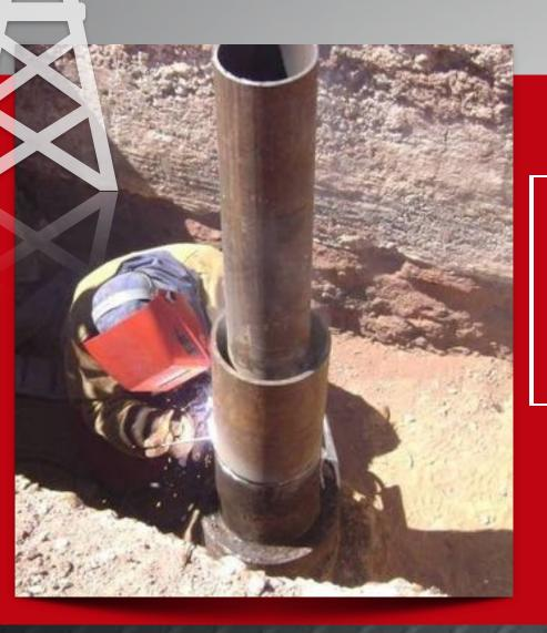
THE 9 5/8" CASING IS EXTENDED AND WELDED IN PLACE ACCORDING TO THE DESIRED HEIGHT PLANNED FOR THE WELLHEAD
