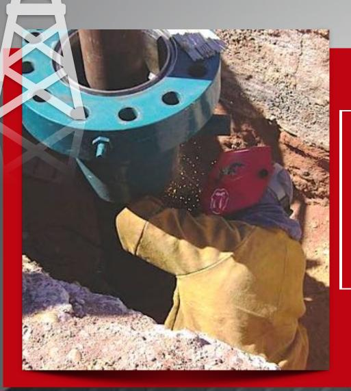
THE 9 5/8" WELLHEAD LEVELLED, THOROUGHLY TACK-WELDED IN PLACE
