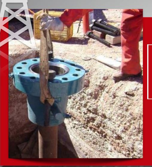
THE 9 5/8" WELLHEAD IS LOWERED ONTO THE 9 5/8" CASING IN PREPARATION FOR WELDING
