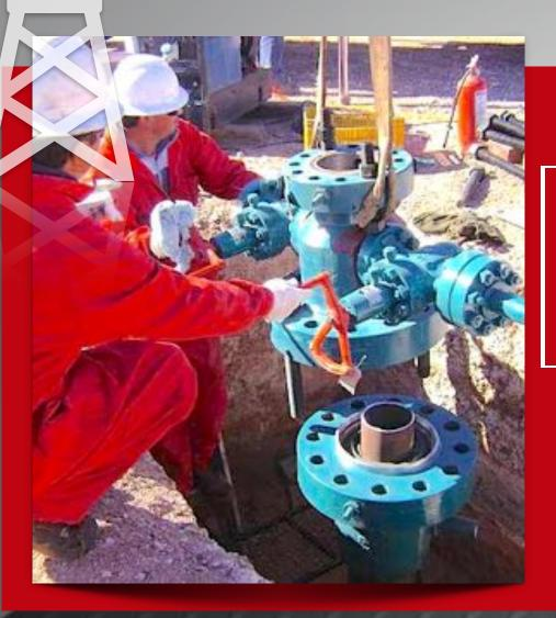
WITH THE PACKER AND STEEL RING IN PLACE, THE 9 5/8" TO 7" REDUCING HEAD IS LOWERED INTO PLACE
