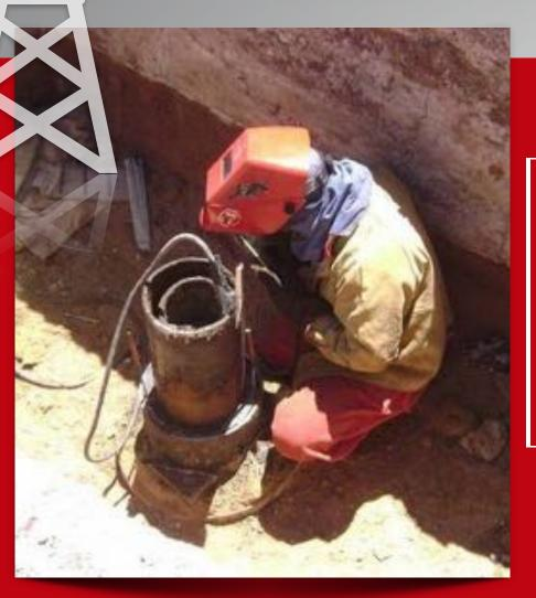
A RING SHAPED PIECE OF FLAT IRON IS USED TO SEAL THE GAP BETWEEN THE TWO OUTER CASINGS
