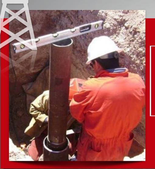
ENSURING THAT THE 7" CASING IS ABSOLUTELY LEVEL IS ESSENTIAL TO THE SUCCESS OF THE EXTENSION PROJECT AS A REDUCER WILL UNITE THE 9 5/8" SECTION AND THE 7" SECTION
