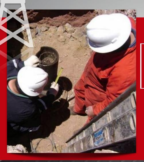
HOT-HED CREWS MARKING THE 9 5/8" CASING FOR THE FINAL CUT
