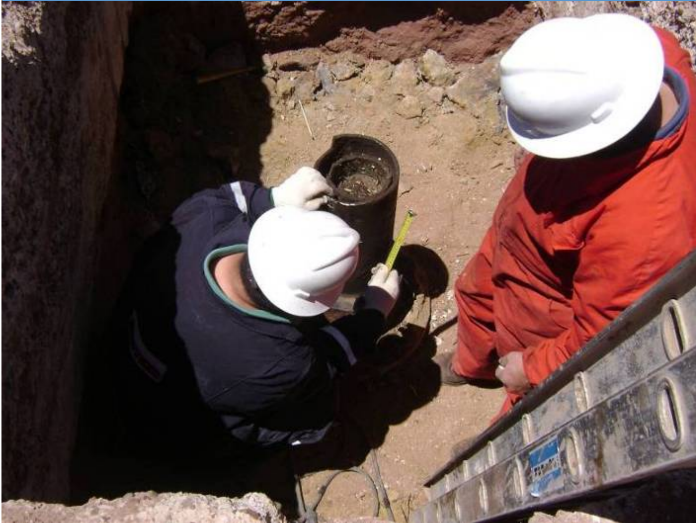
HOT-HED CREW MARKING THE 9 5/8" CASING FOR THE FINAL CUT
