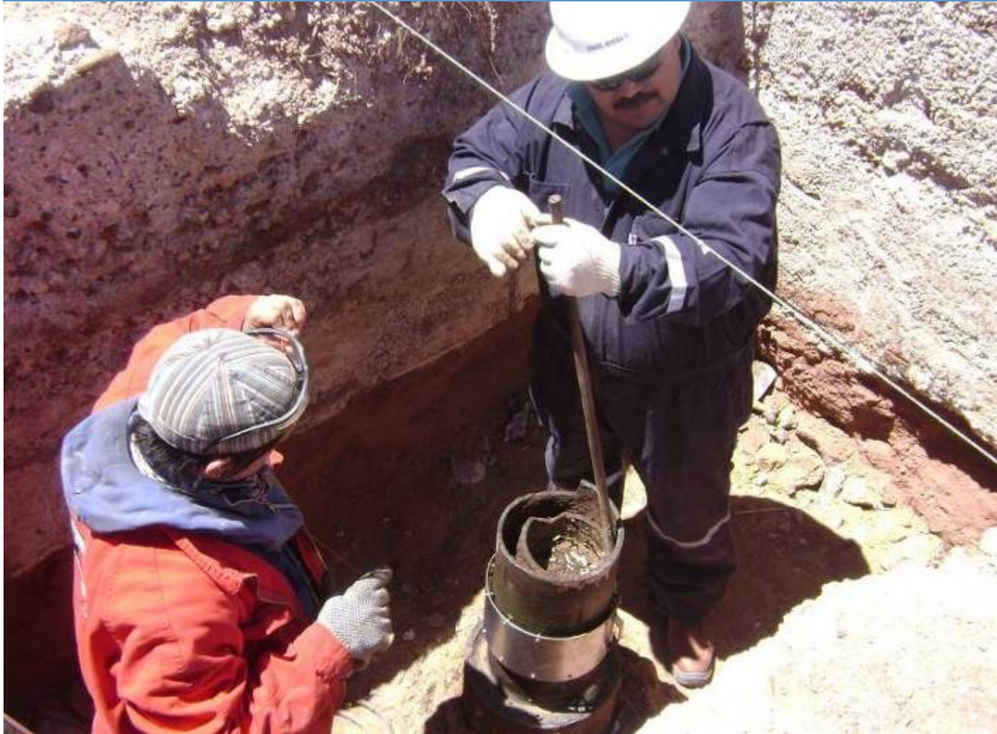
HOT-BEVL'R BEVELING BAND IN PLACE WHERE CUT WILL BE MADE
