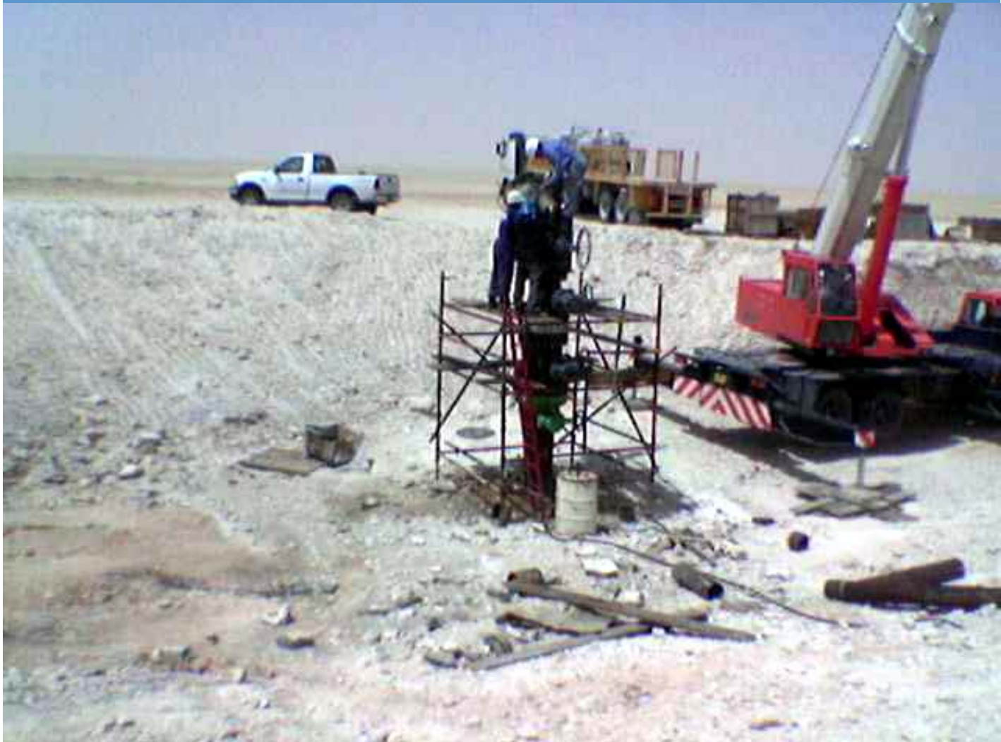
FINAL HYDRAULIC PRESSURE TEST
